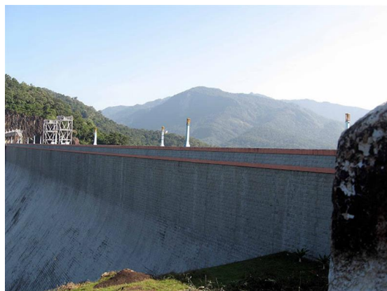
View of Downstream face of the Dam
